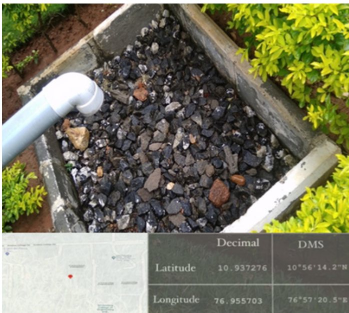
Rainwater harvesting pit & Runoff collection Pond
