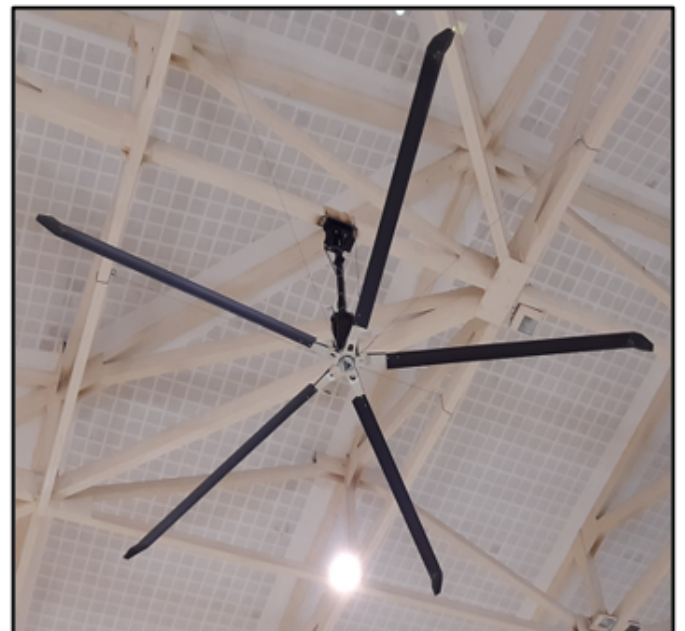
High Volume Low Speed (HVLS) Fan 2HP, 3 Phase Motor, Speed of 80 rpm HVLS fan at Vankatram Learning Center (Library) and Sri Krishna Hall
