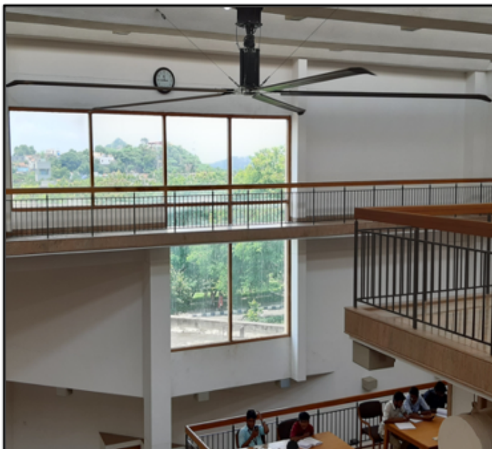
High Volume Low Speed (HVLS) Fan 2HP, 3 Phase Motor, Speed of 80 rpm HVLS fan at Vankatram Learning Center (Library) and Sri Krishna Hall
