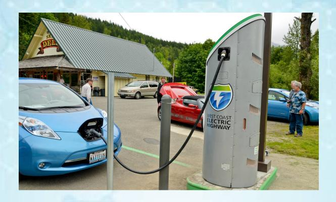
An electric vehicle charging station, also called EV charging station, electric recharging point, charging point, charge point, ECS (electronic charging station), and EVSE (electric vehicle supply equipment), is an element in an infrastructure that supplies electric energy for the recharging of plug-in electric vehicles including electric cars, neighborhood electric vehicles and plug-in hybrids.
