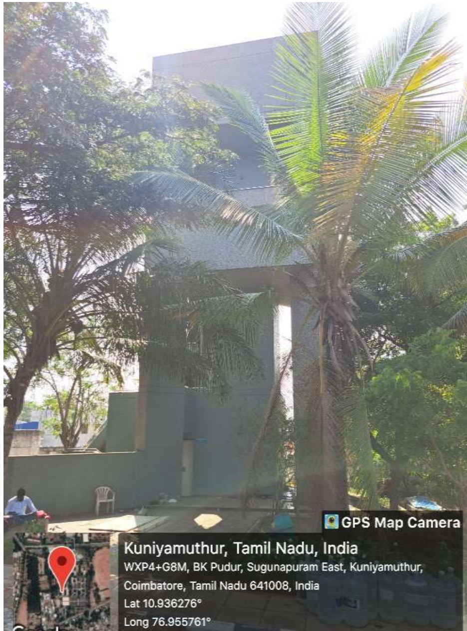
Overhead Water Tank
