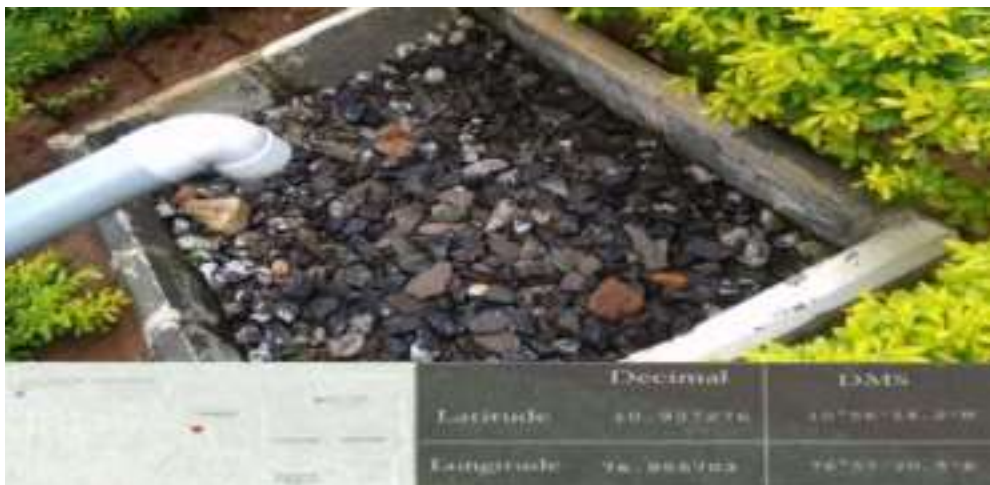
Rainwater harvesting pit (Top view)
