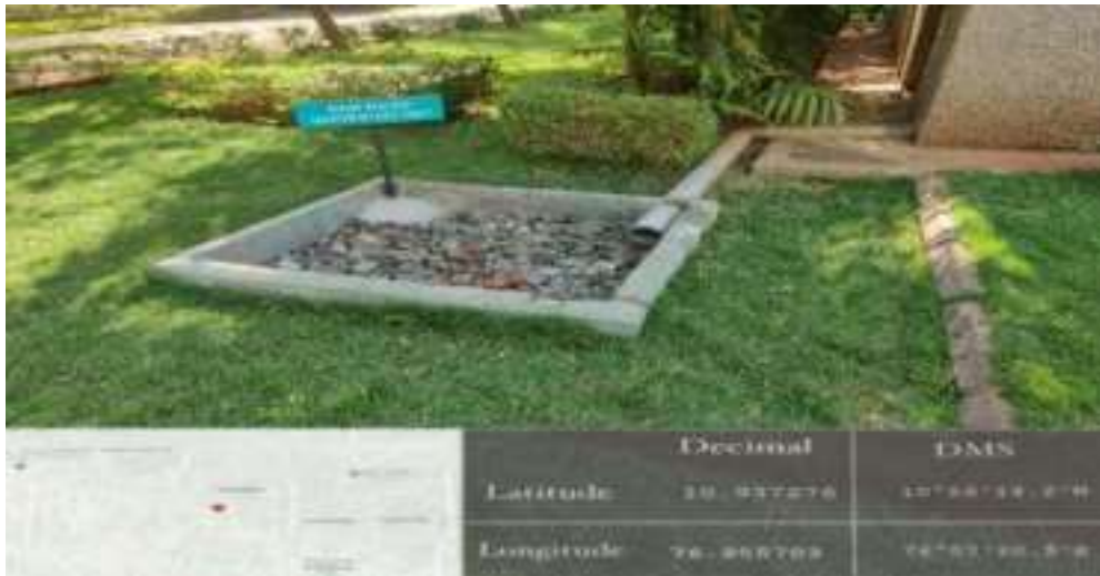
Rainwater harvesting pit (Long view)
