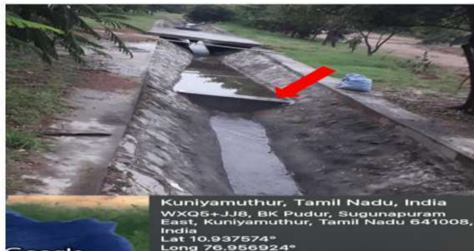
Check dam along the runoff channel with percolation pits (Rainy Season)
