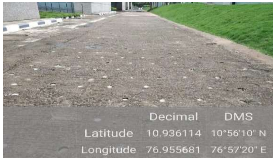
Perforated drain channel slabs (Long view)
