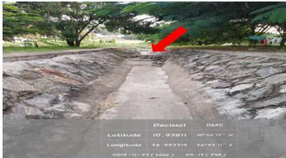
Check dam along the runoff channel with percolation pits (Dry Season)
