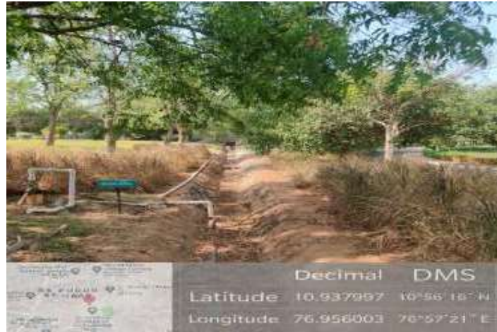
View of the bore well recharge facility
