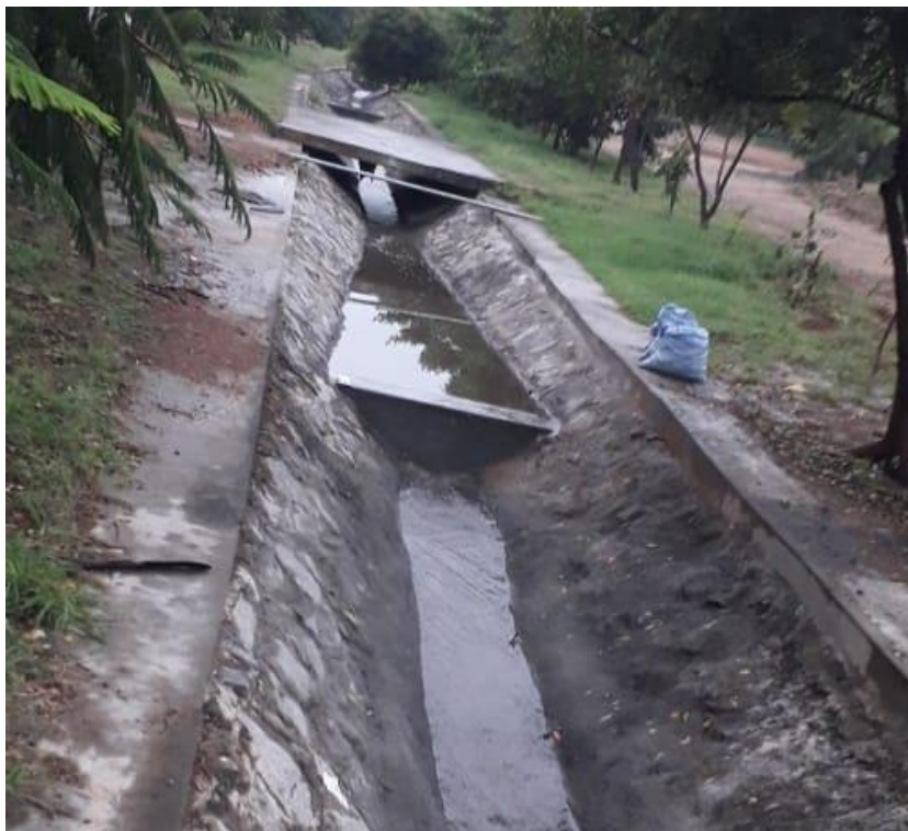
Percolation pits by deep bore holes (Rainy Season)
