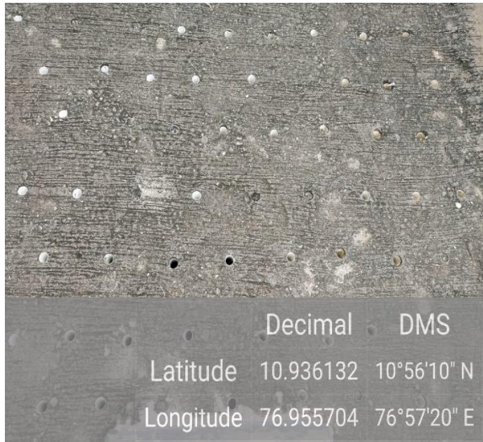
Perforated Drain Channel Slabs (Close view)
