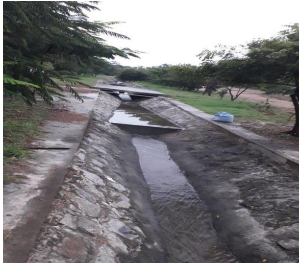
Percolation pits by deep bore holes (Rainy Season)
