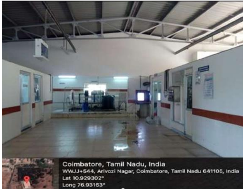
RO plant front view
