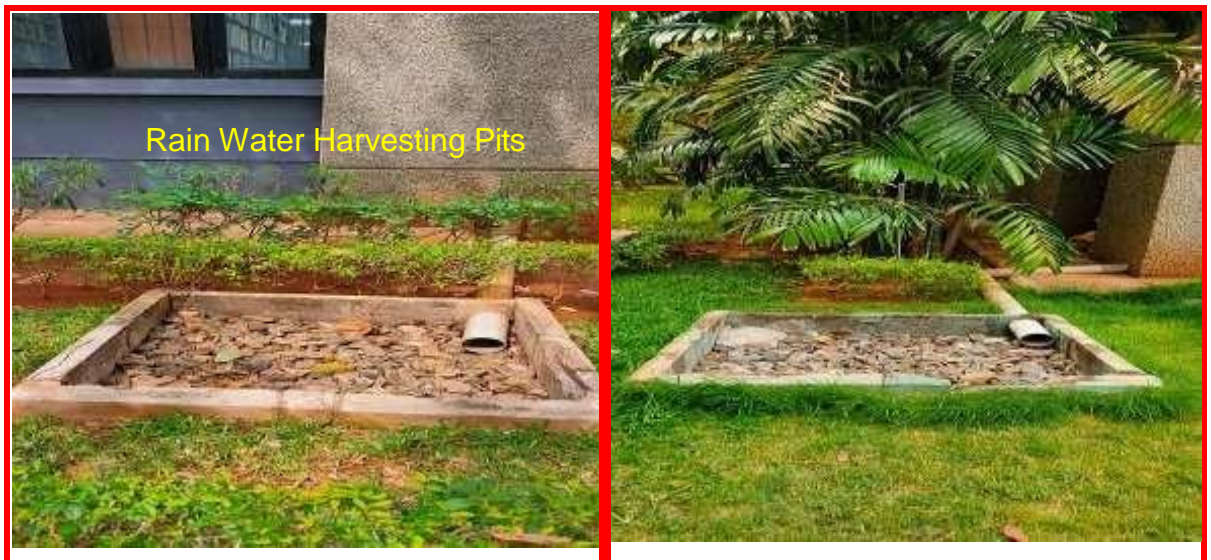
Building Roof Run off based Rain Water Harvesting System
