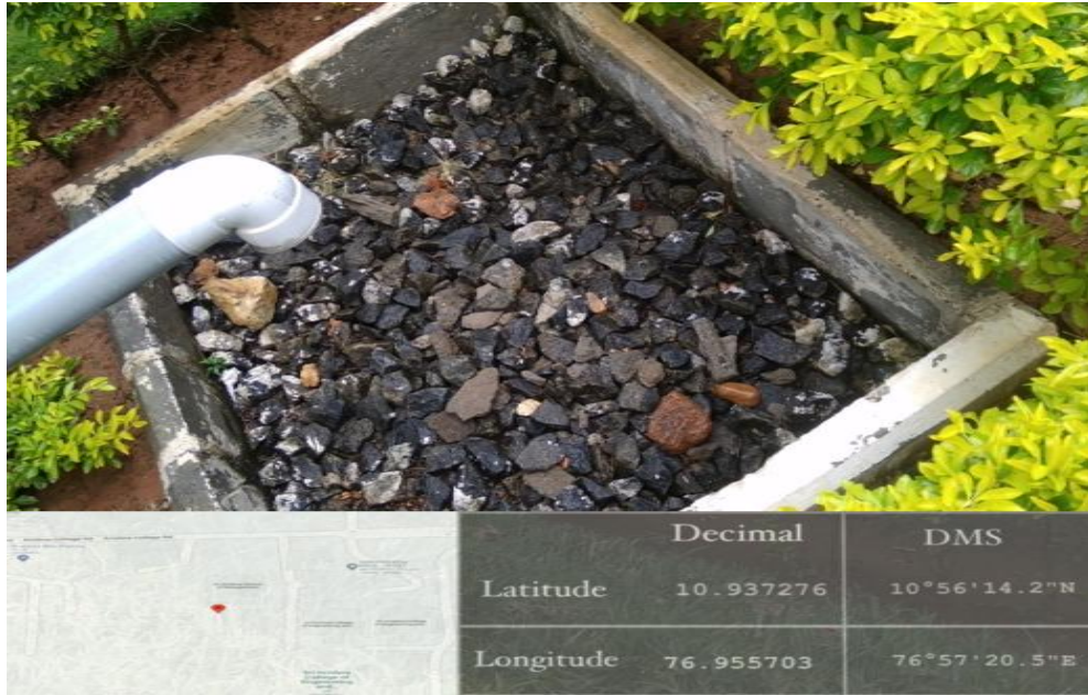
Rainwater harvesting pit (Top view)
