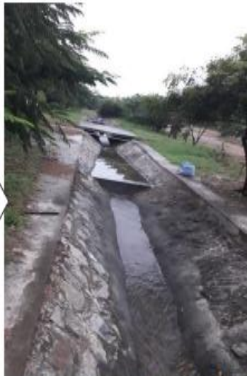
CHANNEL WITH CHECKDAM
