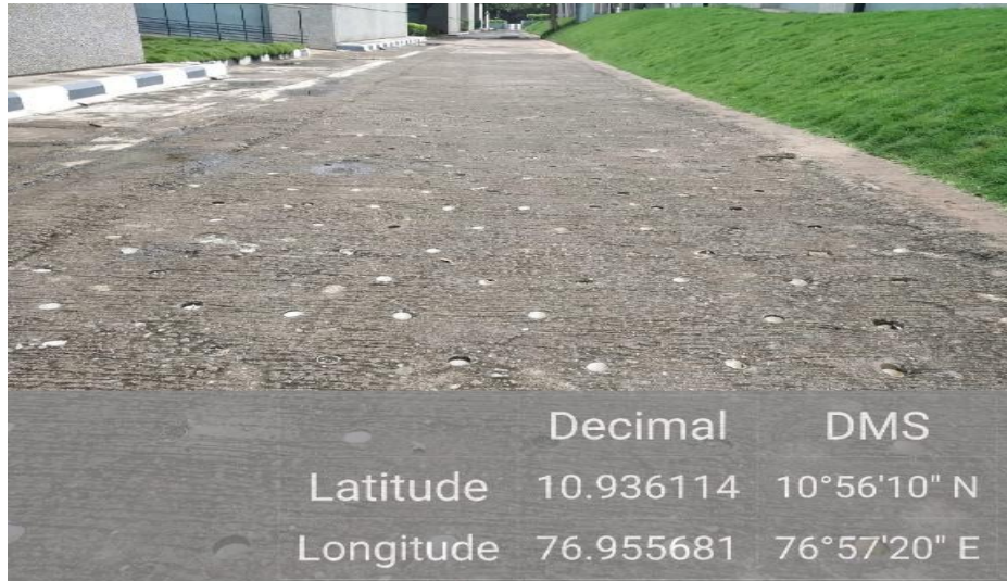
Perforated drain channel slabs (Long view)
