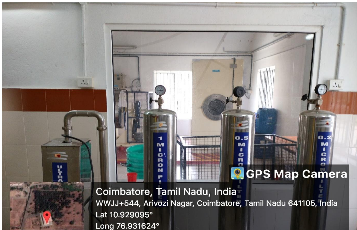
Filtration units inside RO plant
