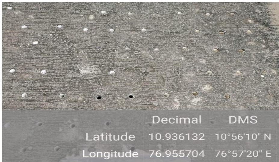
Perforated drain channel slabs (Close view)
