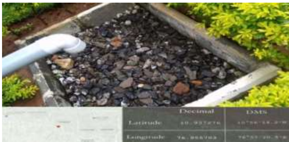
Rainwater harvesting pit (Top view)
