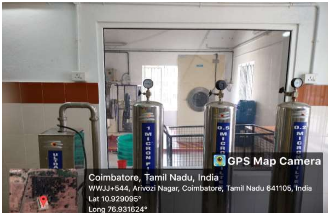
Filtration units inside RO plant
