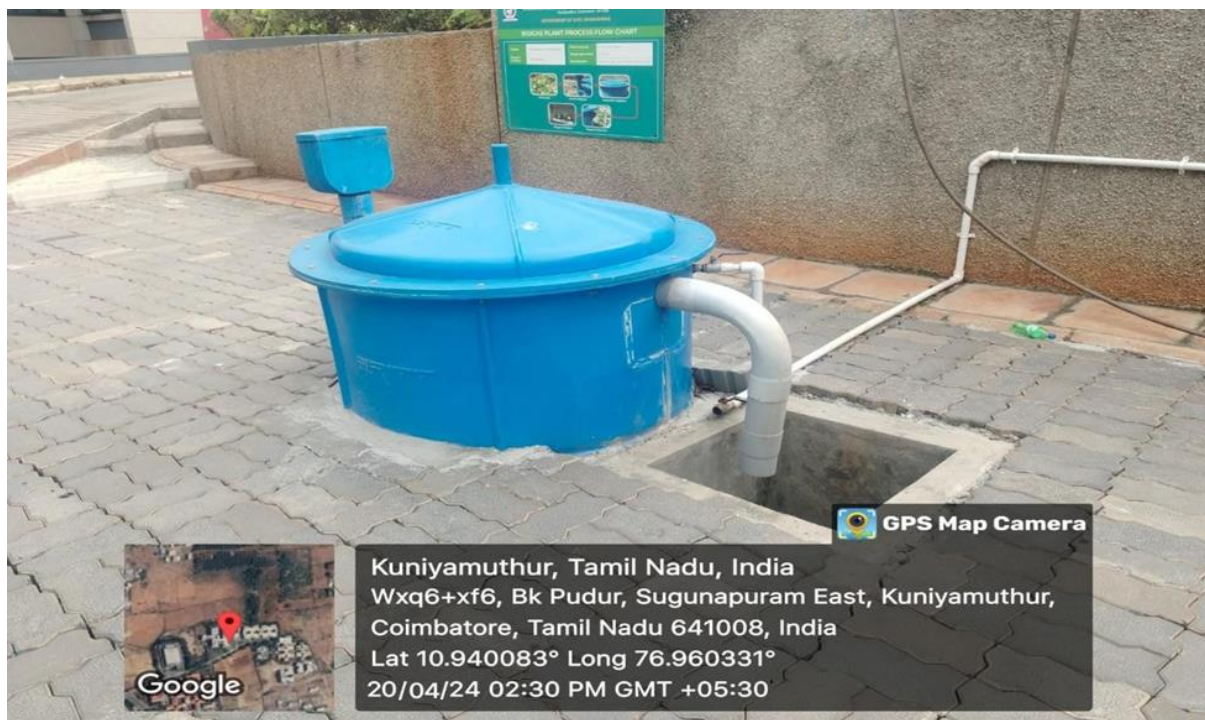
Bio gas Digester with 2 Cubic meters Capacity and Gas 1 Kg/Day
