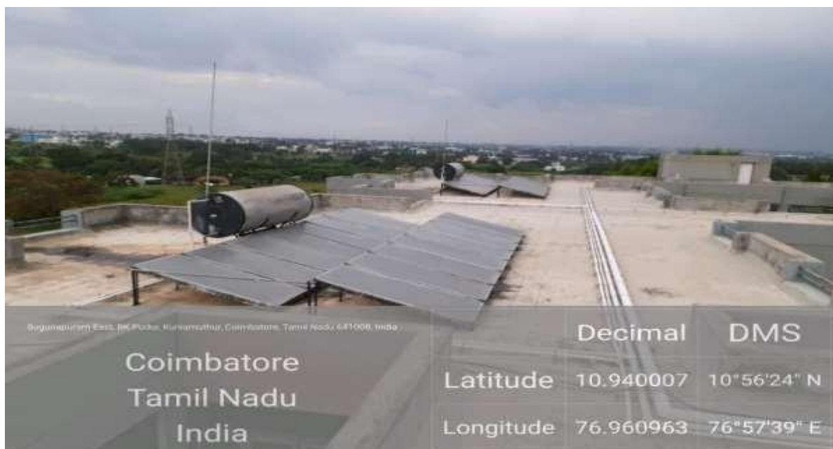
Solar water heater installed in Hall of Residence Women-'B2' Block 3000LPD with 5bar(kg/cm 2 )
