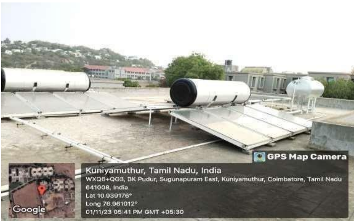
Solar water heater installed in Hall of Residence Men –‘C’ Block 3000LPD with 5bar(kg/cm 2 )
