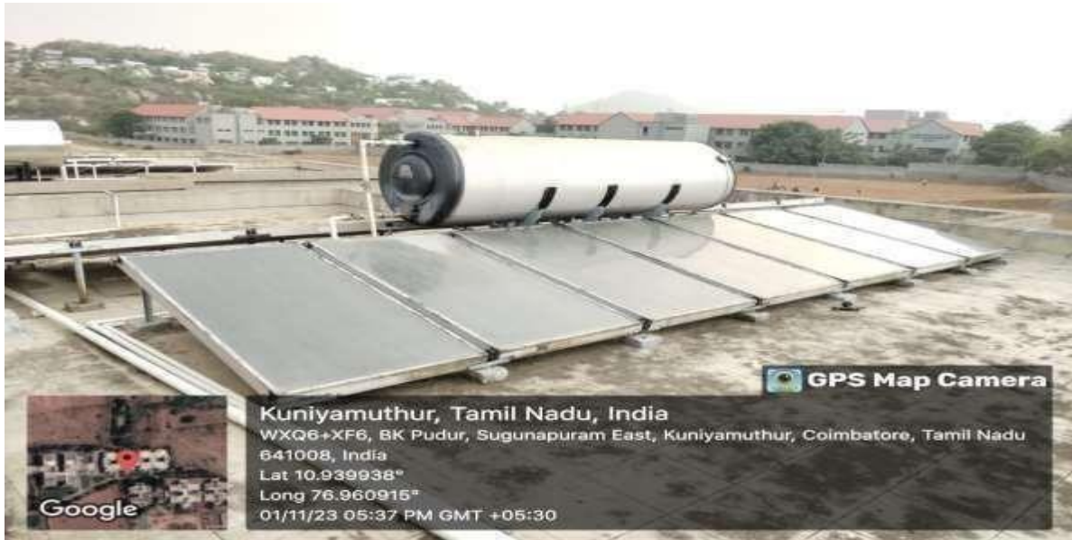
Solar water heater installed in Hall of Residence Men –‘C’ Block 3000LPD with 5bar(kg/cm 2 )
