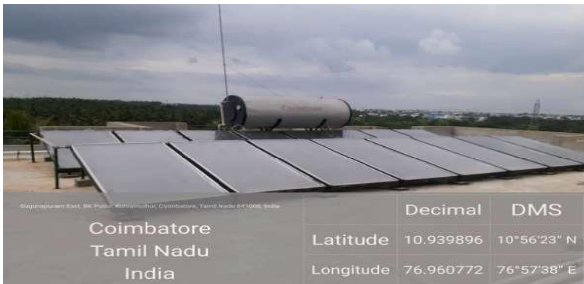
Solar water heater installed in Hall of Residence Women-'B1' Block 3000LPD with 5bar(kg/cm 2 )
