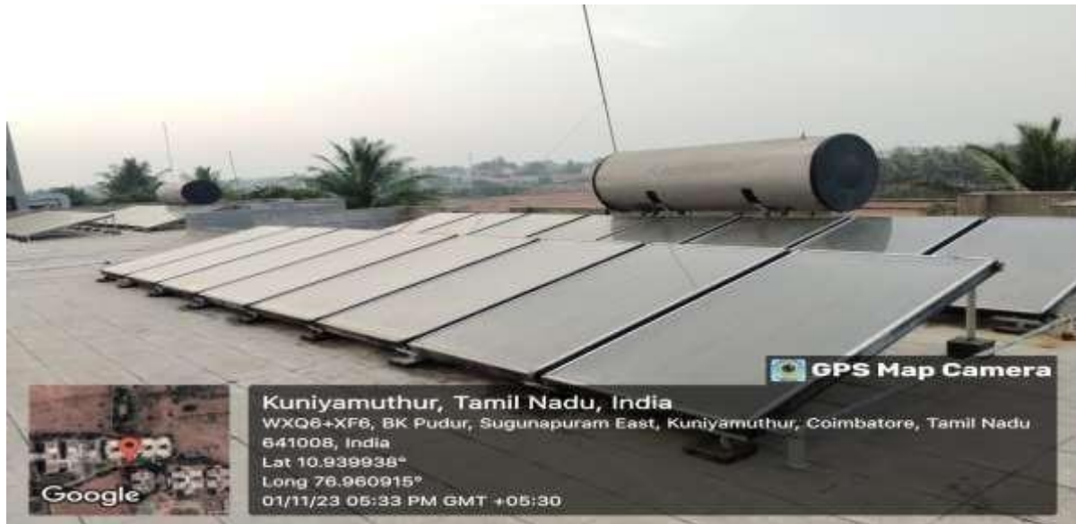
Solar water heater installed in Hall of Residence Men –‘A’ Block: 3000LPD with 5bar(kg/cm 2 )
