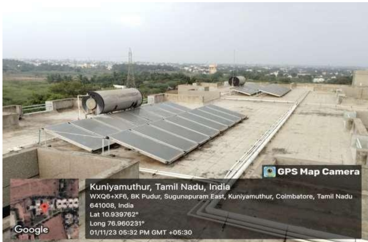
Solar water heater installed in Hall of Residence Men –‘B’ Block 3000LPD with 5bar(kg/cm 2 )
