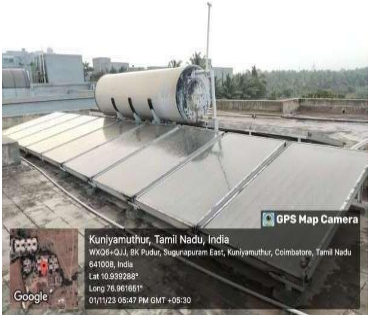
Solar water heater installed in Hall of Residence Men –‘E’ Block 3000LPD with 5bar(kg/cm 2 )
