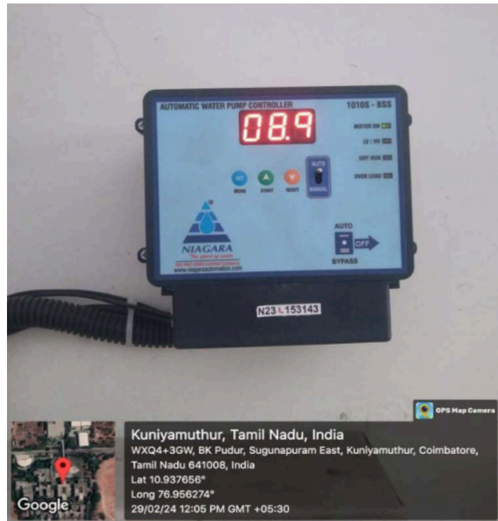
Automatic Water Pump Controller – Administrative Block
